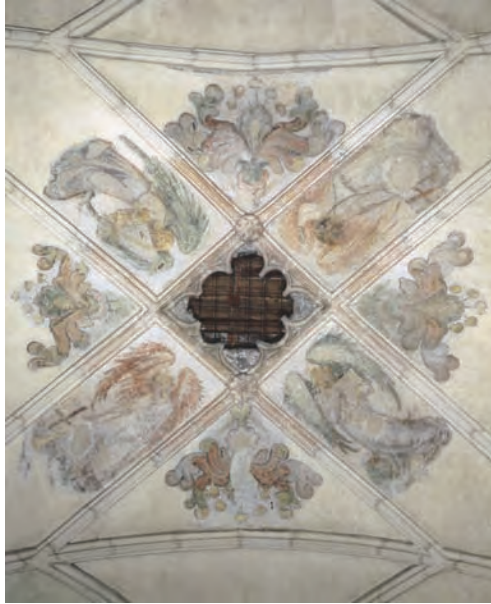
Illustration 14. An Opening in the Church Nave for Pulling in the Statue of the Resurrected Christ. St Nicolas Church in Znojmo. Reproduction: Kaliopi Chamonikola (ed.). Od gotiky k renesanci. Výtvarná kultura Moravy a Slezska 1400-1550 II . Brno, 1999: 213.
