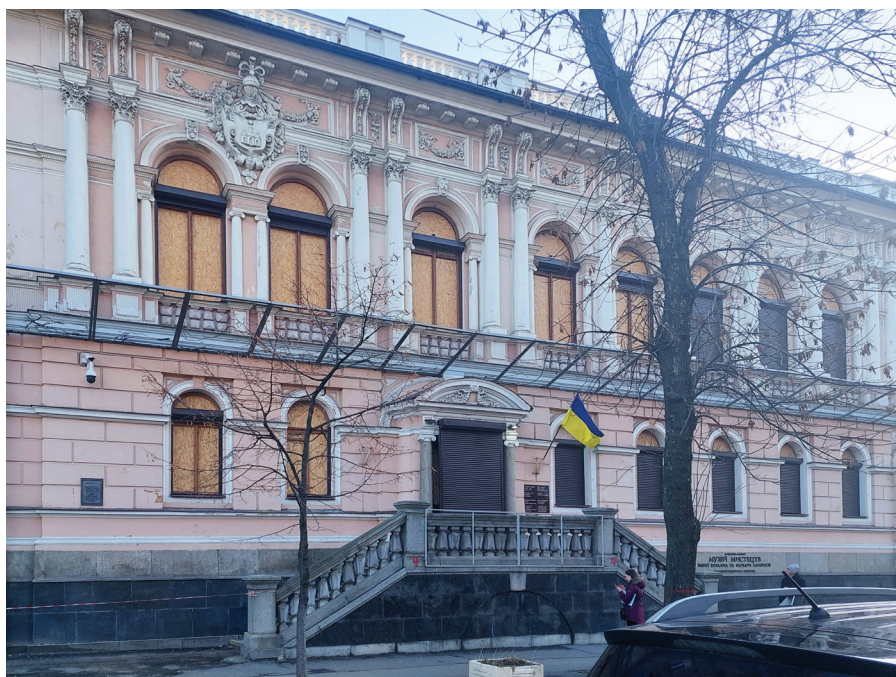
Fig. 1: The facade of the Bohdan and Varvara Khanenko National Art Museum with boarded up windows (Photo: Y. Ivashko, 2024)
