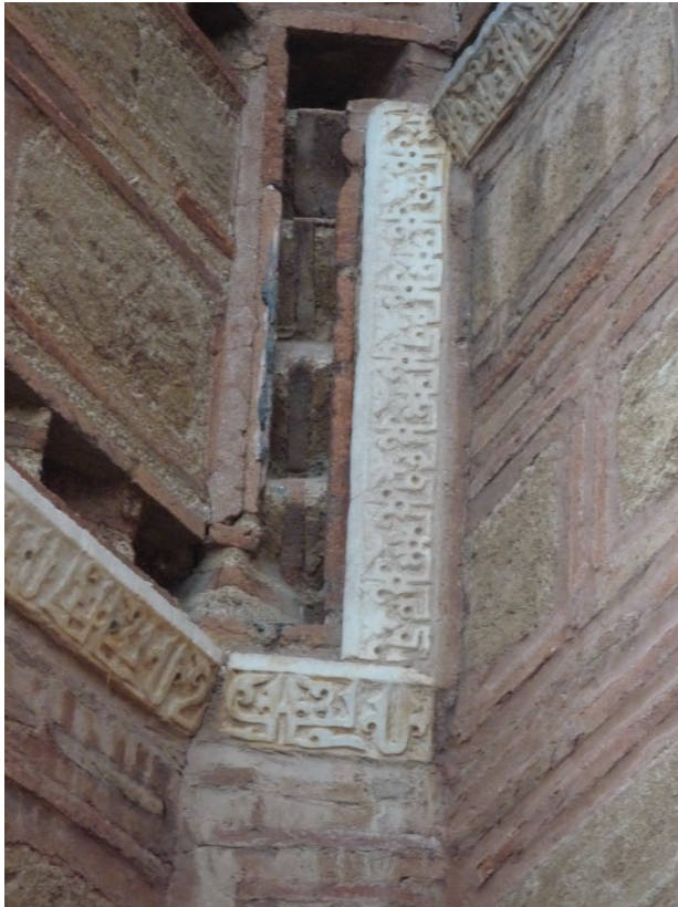
2 – Champlevé cornices , 10 th century. East side of the Panagia Church, Hosios Loukas Monastery
