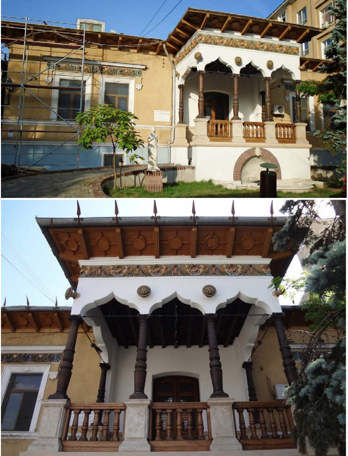
Figure 7: Ion Mincu, Lahovari House, Bucharest, 1886. Front façade / detail with the front porch.
