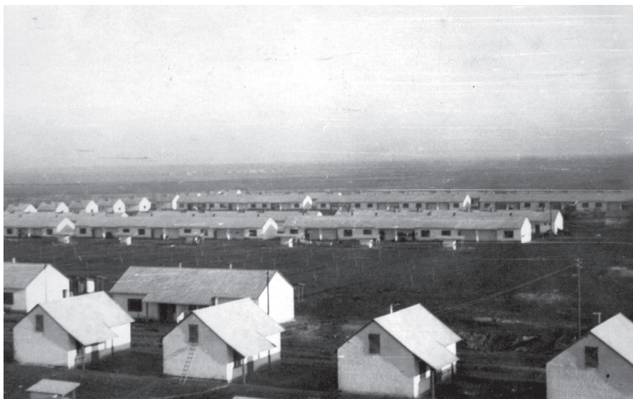
Figure 6. The Greek village under construction. © Vlachos – Raptis – Fokas (eds.) 2017.
