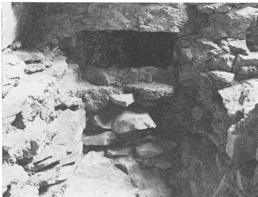
Fig. 4. – East side of the trench with partly opened grave pit. The difference between the grave-pit mortar and "Romanesque mortar" may be clearly seen in front of the picture at the aperture. Photo by V. Jílková.
