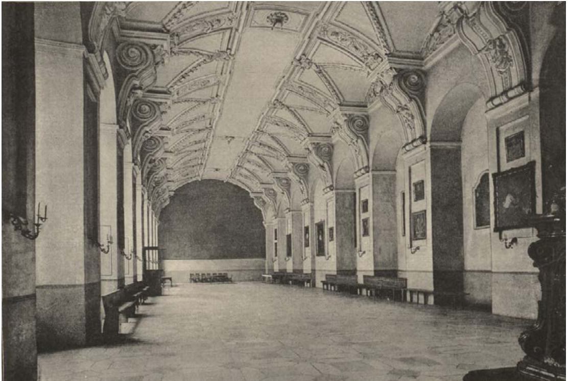
Figure 5: View of the Interior of the Clementinum Refectory, before 1891.
