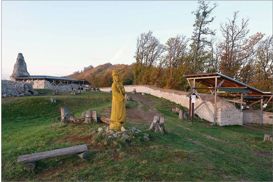
Fig. 4. Deserted Castle in Zvolen, Lower Castle. View from the courtyard at the reconstructed entrance gate, western line of the fortification and the residential tower (in the background on the left), 2019. Photo by Ján Beljak.
